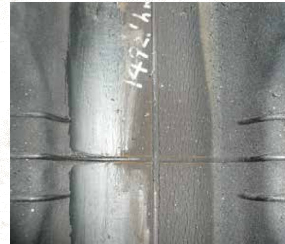
Small ozone cracks
